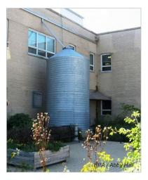
A large cistern collects roof runoff from a commercial building in Chicago.
