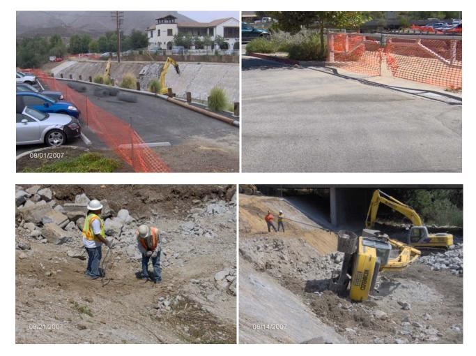
The contractor was very safety conscious. He required his workers to wear safety vests, hard hats and protective gear at all times. However, despite the most vigilant approach to safety, accidents do still occur. In order to remove debris from the channel, a 2 step process was utilized. The lower excavator would place debris in a pile that the upper excavator would then place in the dump truck. In
