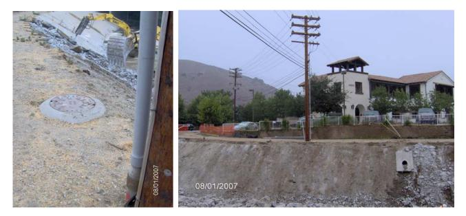
After the concrete removal the sewer line was inspected and it suffered no damage. Fortunately, the power pole was located on the bank and due to its elevation was not at risk of being hit by the excavators that were working in the channel. However, one of the power poles did hamper debris removal because it forced the dump trucks to have to use the downstream entrance, which exited directly onto a busy road.
