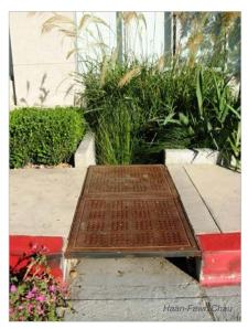
Curb cut that directs water from the street into a bioswale. Voluntarily installed at 1100 S. Hope Street in downtown L.A.
